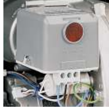
Control box fitted with an ignition transformer
